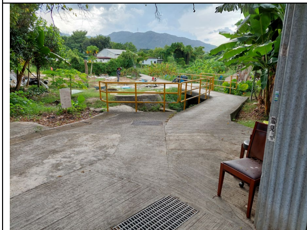
Plate 11 – Existing 750mm U channel receiving discharges from the subject site and running southwestward toward an existing watercourse
