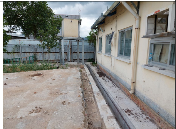
Plate 6 – Existing peripheral 300UC within the western subject site boundary
